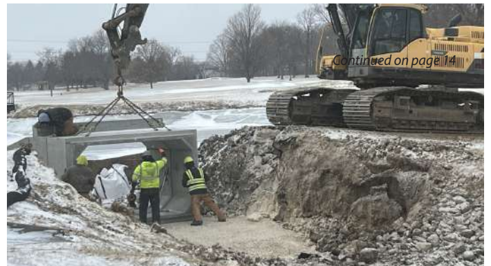
Installation of precast culvert sections.
